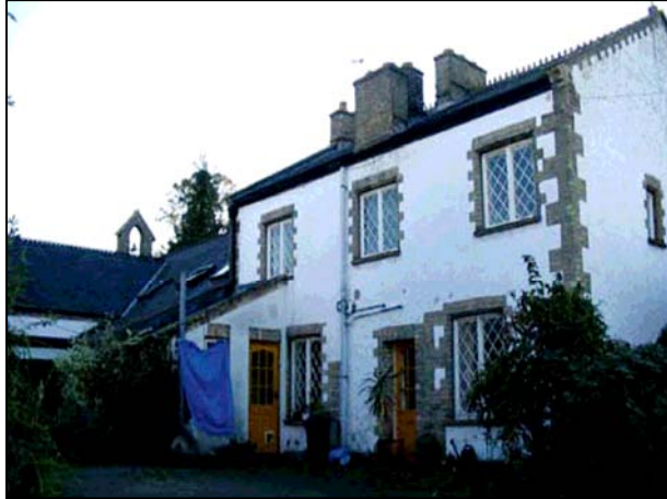
Rear of School House, School Lane
