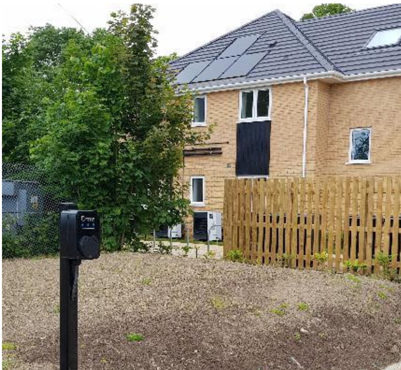
Figure 9: new development at Arbour Sq, with charge point, ASHP (middle of photograph) and solar panels
