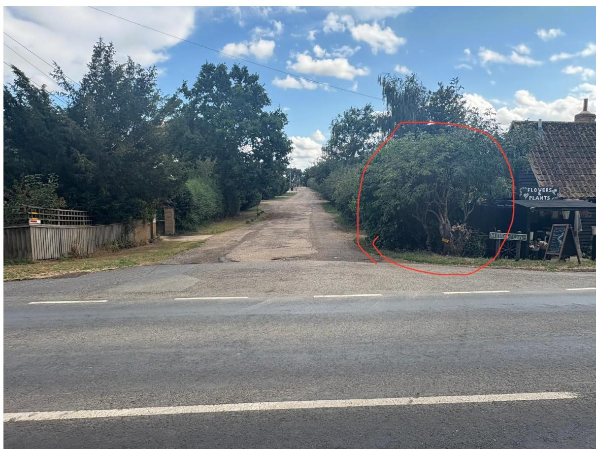
The current width of the lane is 6.1 meters, (although the width of a road will depend on purpose and location, rural road are generally 5.5- 6 meters)
