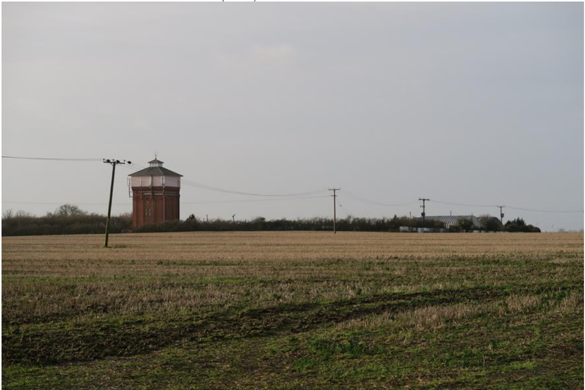
Picture 11: View of Soham Water Tower (FV07)
