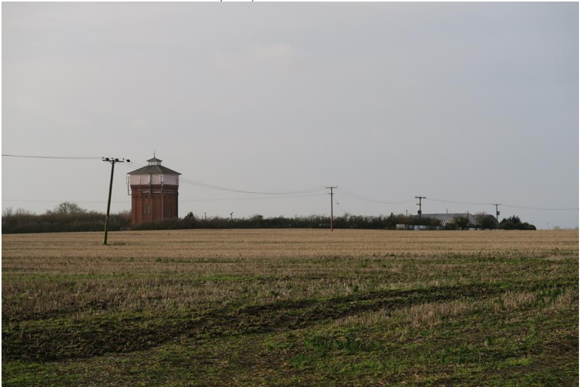
Picture 11: View of Soham Water Tower (FV07)
