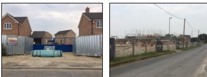
Image 8: New homes currently under construction on Fordham Rd Isleham
