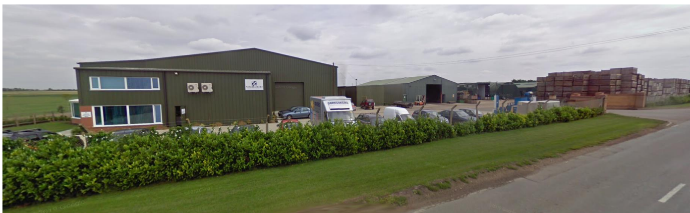
Westmoor Common – Farm buildings within the proposed site.
