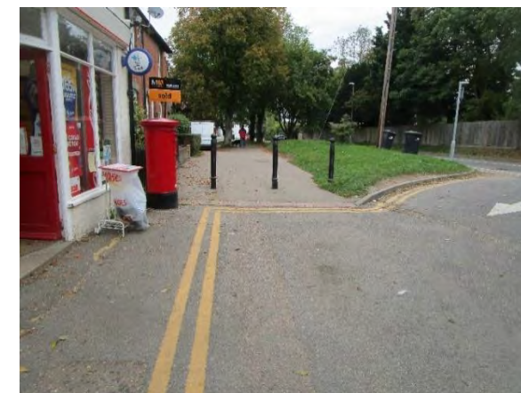
For the link with Parsonage Road access to this area from The Causeway needs to be closed off.
