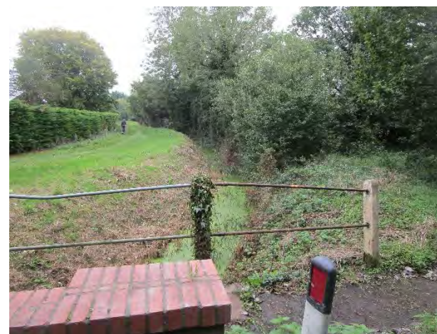
View along Catch Water Drain from Station Road. This is private land and any route that can be agreed would be likely to follow field boundaries and water courses and would need to allow for farm vehicles.
