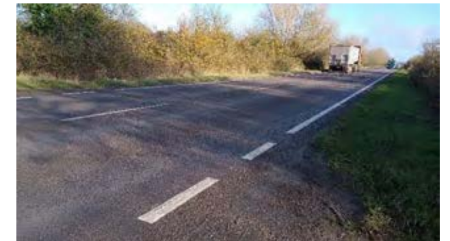
Figure 7A.18.2 The A142 crossing.
