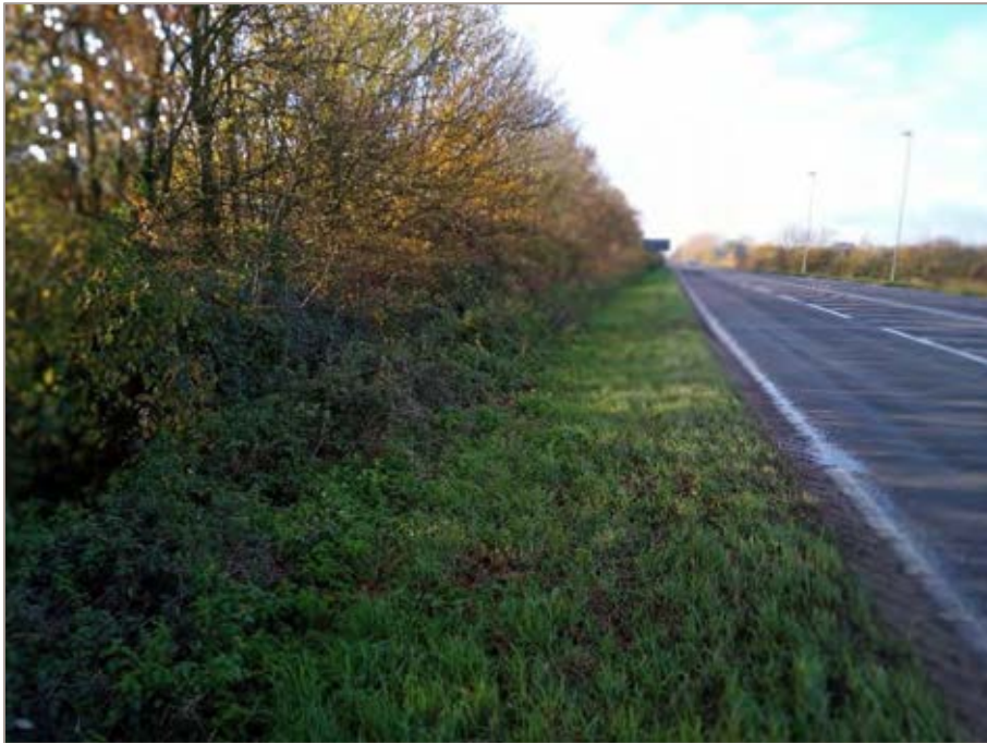
Figure 7A.21.3 View along A 142 verge, where a 4m ramp would need to be. It would need to be set back from the road so would impact on trees and a ditch to the left.
