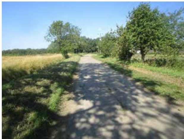
Figure 7A.15.1. Road by Common Farm.
