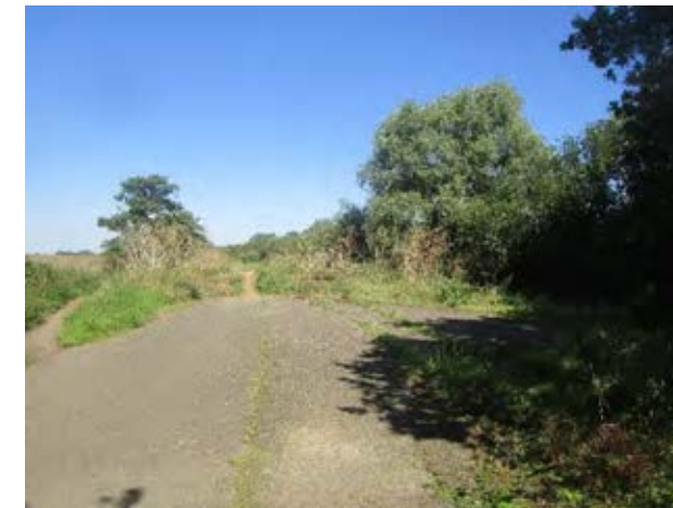
Figure 7D 4.2 Mepal Road showing earth piled across the road.
