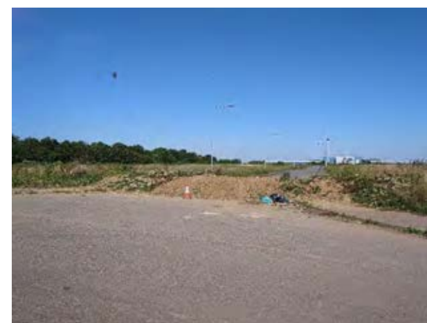
Figure 7B 6.1 The existing road infrastructure in Elean Business Park does not include cycling provision crossing, which needs adding with segregated cycleways and segregated footways.
