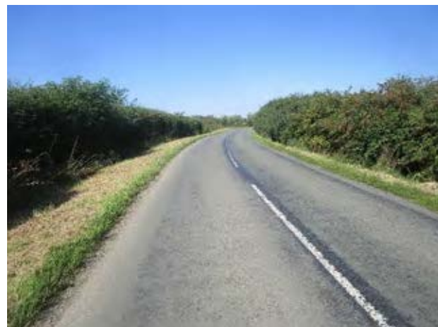
Figure 7A.2.1 Mepal Road. The centre lines suggest high speeds may be appropriate.
