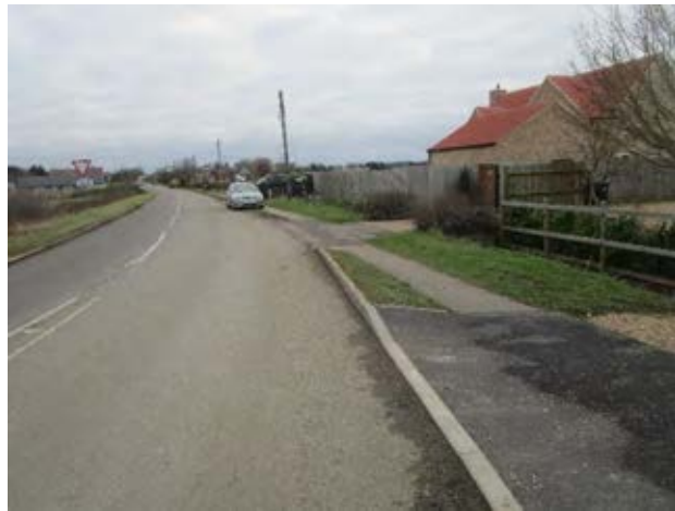
Figure 7B 16.1 This section of road on the edge of Witchford either needs to be 20 mph with carriageway changes for cyclists to mix with traffic or a widened and extended shared use path is needed on the right with carriageway narrowing and a 30mph limit.
