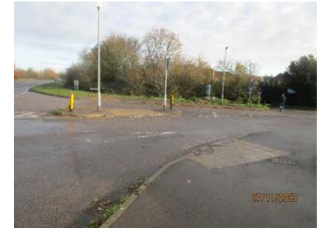
Figure 7AE 32.1 Current crossing provision does not comply with LTN 1/20 and is not suitable for all.
