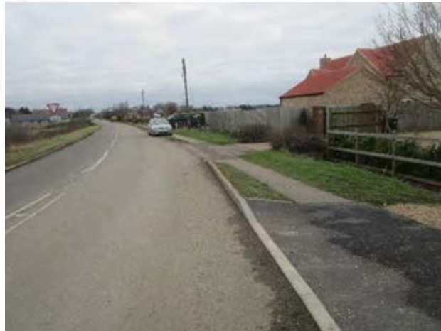
Figure 7C 15.1 This section of road on the edge of Witchford either needs to be 20 mph with carriageway changes for cyclists to mix with traffic or a widened and extended shared use path is needed on the right with carriageway narrowing and a 30mph limit.
