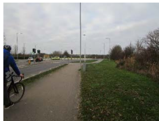
Figure 7C 4.3 The existing Lancaster Way crossing of the A142.
