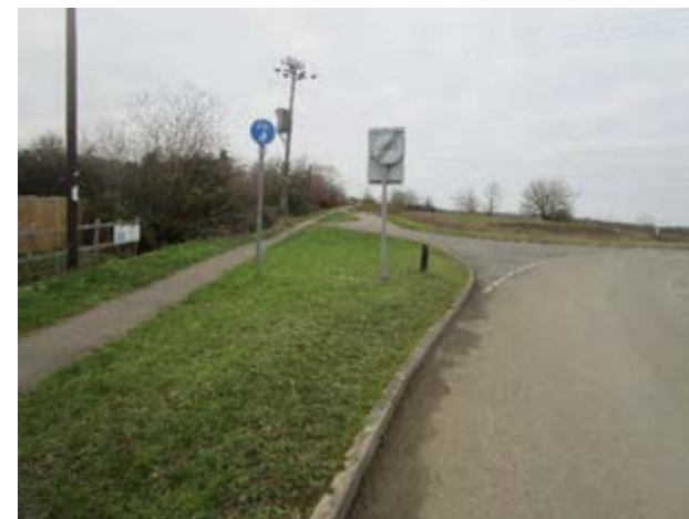
Figure 7B 15.1 The route could either use the existing path to the left or a new ramp and bridge linking to the land on the right.
