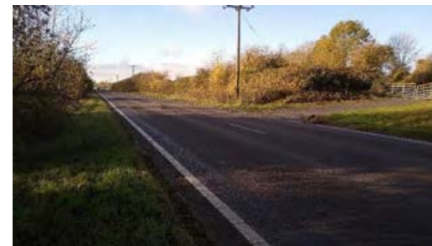
Figure 7B 19.1 A142 with byway/ farm access on the right and overhead lines just visible.
