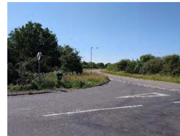
Figure 7A.1.4 Witcham Road/ Sutton Road junction that needs modifying.
