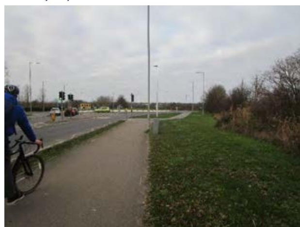
Figure 7B 4.2 The existing crossing in a similar location by Lancaster Way .
