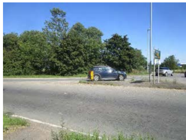
Figure 7C 4.1 Existing crossing provision is inadequate.
