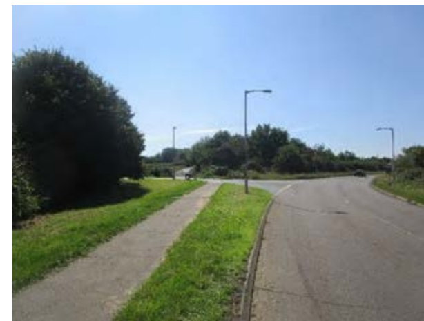
Figure 7A.1.3 Witcham Road/ Sutton Road junction that needs modifying.
