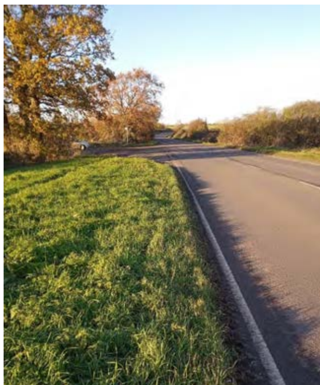
Figure 7D 12.1 View of the potential crossing point along the A1421 with the bridleway starting where the car is parked on the left and the road bending to the right beyond.
