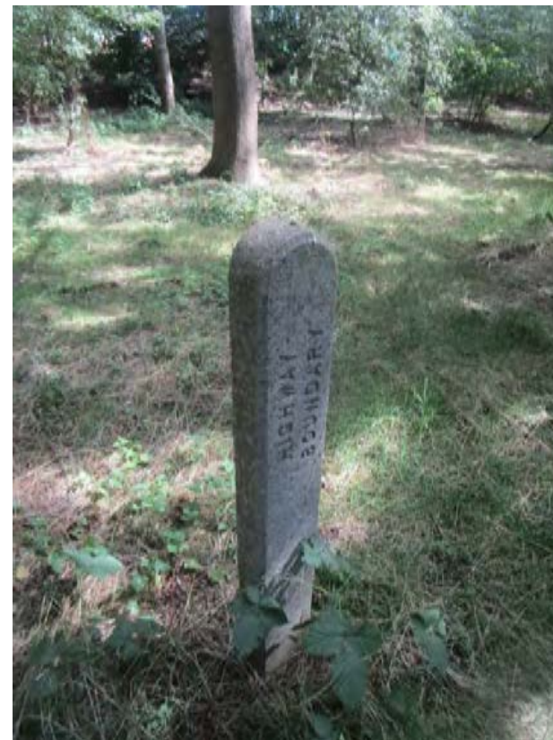
Figure 7B 3.5 Highway boundary markers show that highway land extends into the woodland, but agreement will also be needed with landowners
