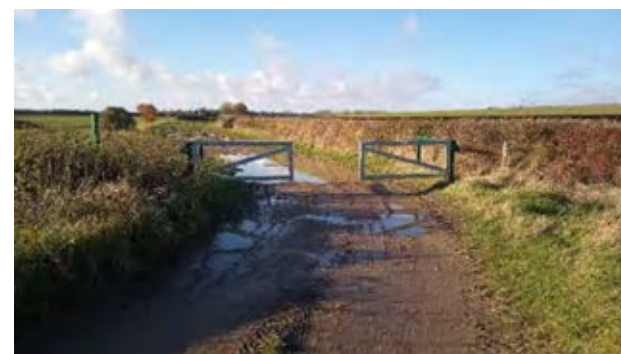
Figure 7B 11.7 Eastern end of byway looking towards Witcham from road in autumn.
