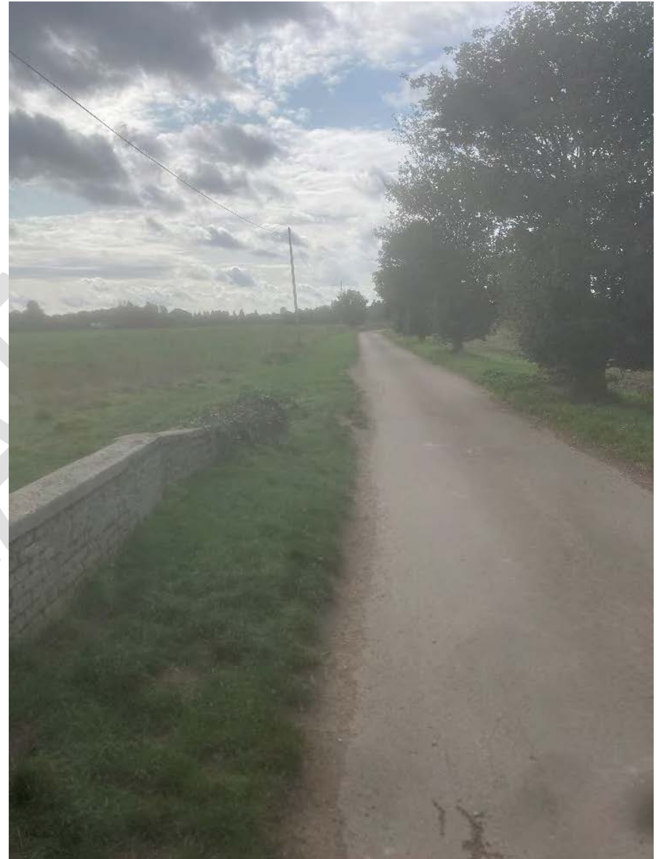
Figure 6.6.2 – River Snail bridge deck (Fordham Moor)
