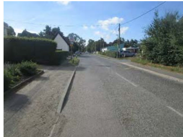
Figure 7A3.1 – View of Isleham Road away from Fordham Primary School.
