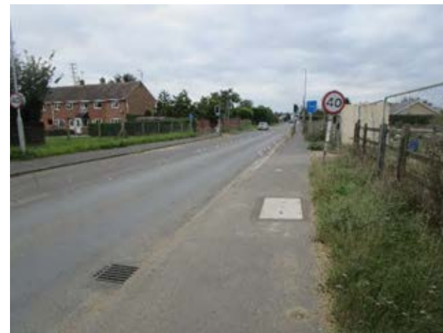
Figure 7E 13.1 View showing narrow path and approach to toucan crossing.
