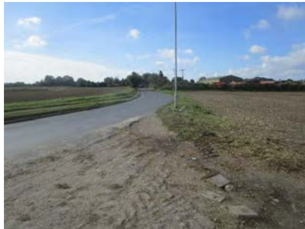
Figure 7A4.1 – View of Isleham Road with existing footway.
