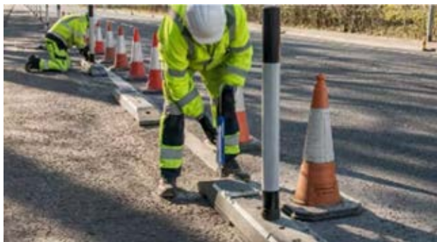
Figure 7A1.3 – Rosehill Highways showing segregated cycleway being established on existing carriageway
