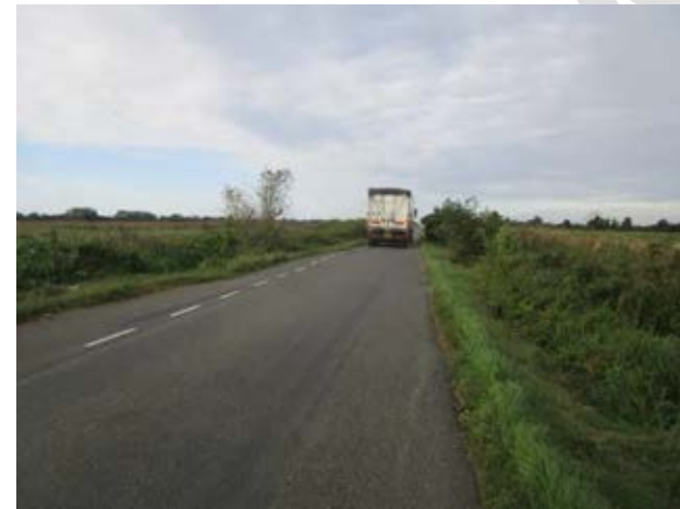
Figure 7E.2 HGV traffic on East Fen Drove
