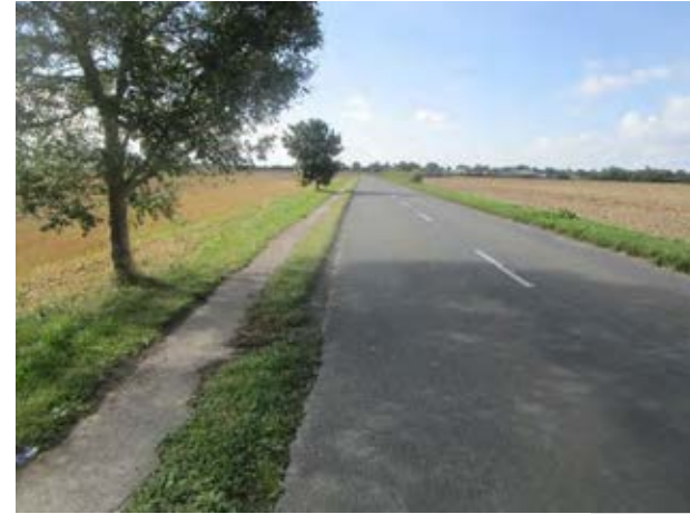
Figure 7A5.1 View towards Fordham with footway on left.
