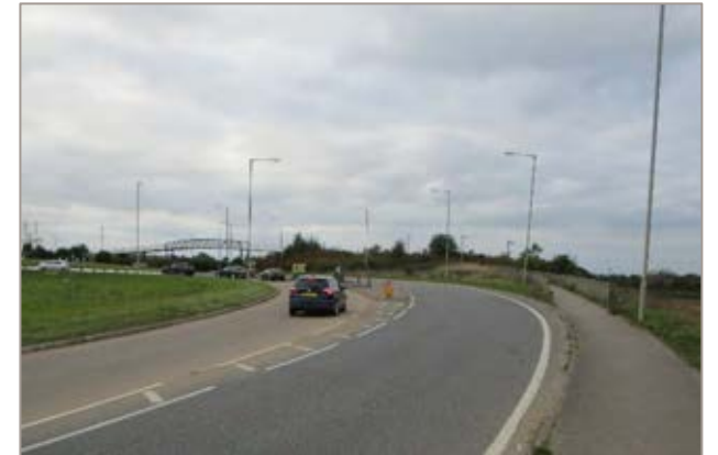
Figure 7E 14.1 View showing the existing bridge and approach ramp.
