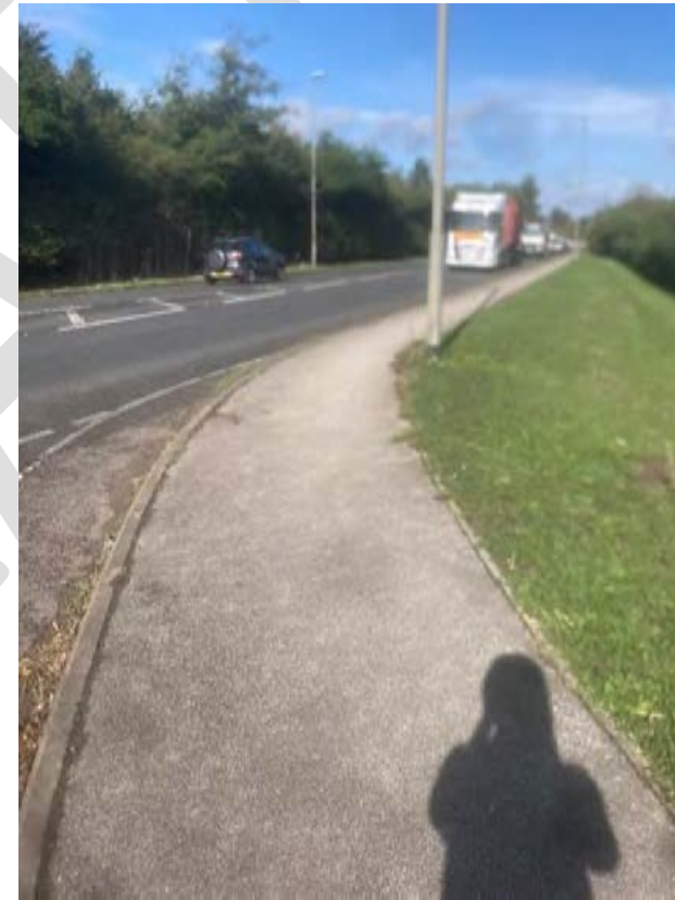
Figure 5.4.2 – Shared use path on Newmarket Road (A142)
