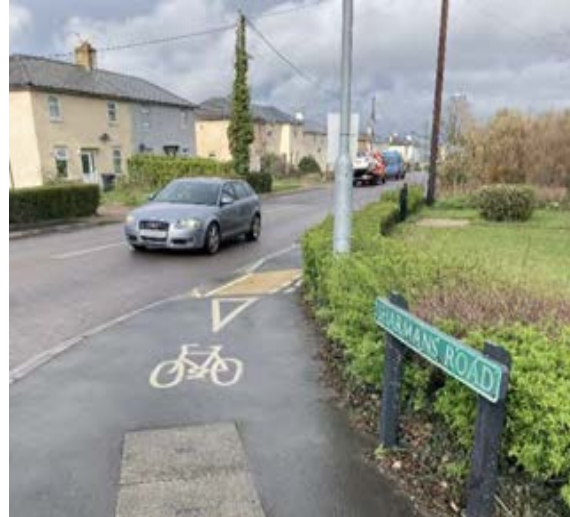
Figure 5.3.2 – Shared use paths in Fordham not compliant with LTN 1/20.
