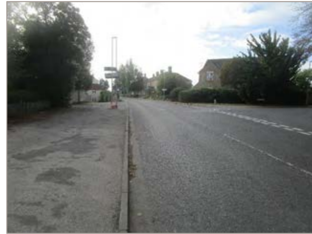
Figure 7A12.3 – Fordham Road/ Mill Street/ Station Road junction where a redesign is recommended to make the junction safer and easier for walking and cycling.
