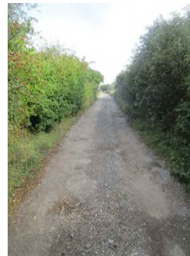
Figure 7A8.2 - Existing access road to Nature Reserve by former railway bridge.
