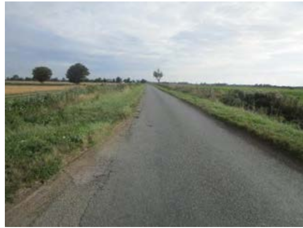
Figure 7E8.1 View along East Fen Drove. The path (vii) would emerge behind the tree on the right and a new path would be needed in the field to the left.
