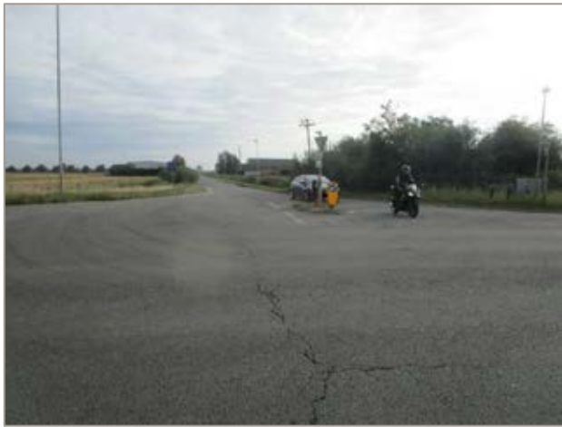
Figure 7E10.1 View from East Fen Common looking across the A142 to East Fen Drove.
