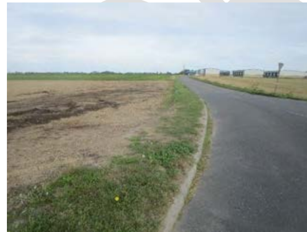
Figure 7A10.1 - View of Hall Barn Road junction.
