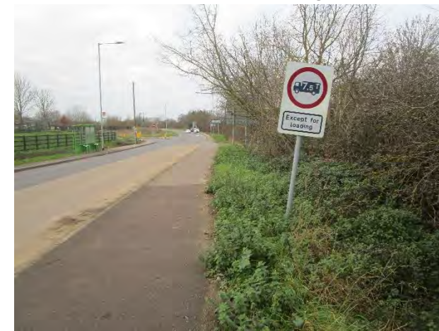
This path is not wide enough and does not have adequate separation from the carriageway and highway space needs reallocating.
