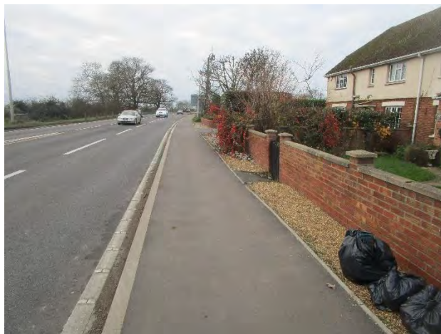
This path is not wide enough and does not have adequate separation from the carriageway and highway space needs reallocating.
