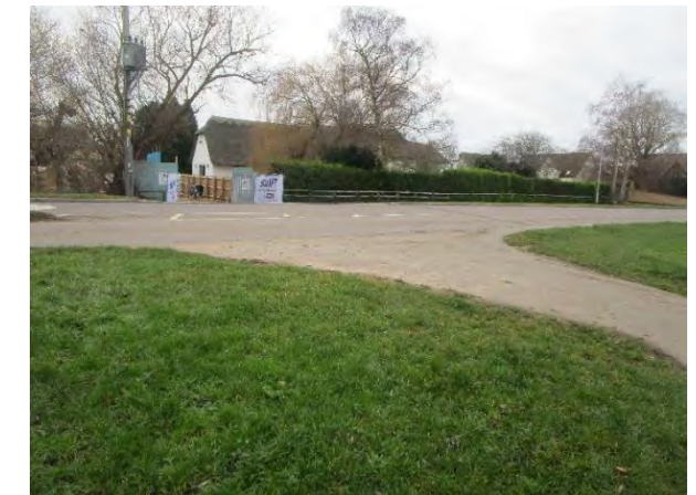
At this location the central island needs removing and a smooth transition is needed between the on-road and off-road routes. Careful design is needed to amend the existing gateway.
