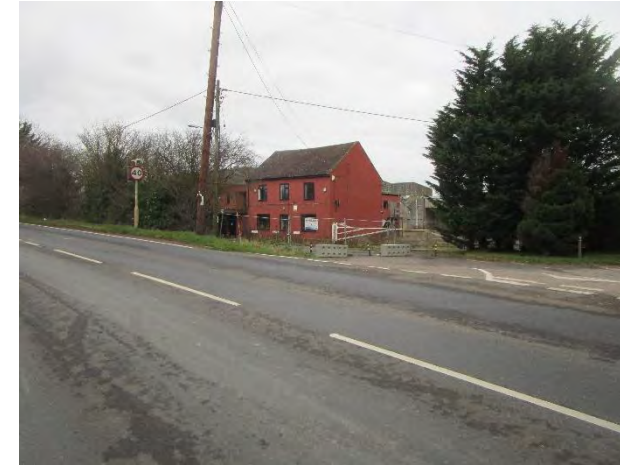
View of A1421 showing limited space available.
