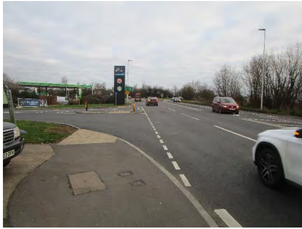
These crossings near the A10 need major changes.
