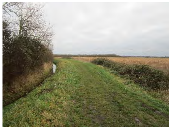
In this location there does not appear to be space for a 3m wide path, so the bank will need widening and additional material will need to be brought in or dug locally.
