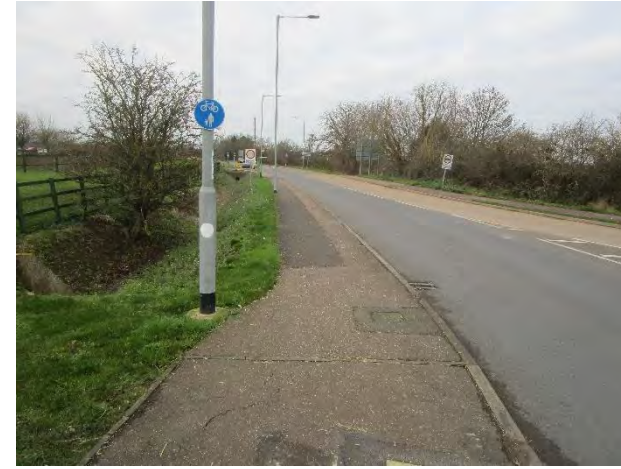
This path is not appropriate as a shared path and should be a footway only, with a cycleway on the other side of the road and new crossings.
