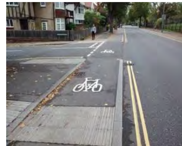
Figure 2: At grade crossing of side road with separation for traffic, cyclists and pedestrians
