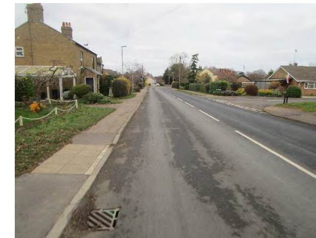
View of A1421 showing limited space available.
