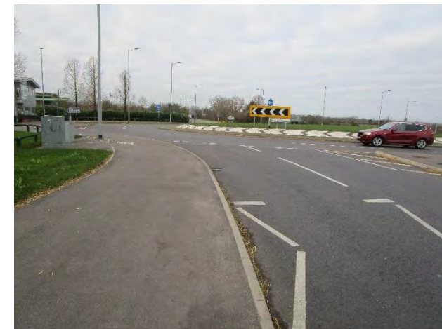
This path is not wide enough and does not have adequate separation from the carriageway. It could be widened, highway space could be reallocated.
