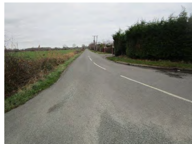
View towards Wentworth from Ely Way/ Church Road/ Pools Road junction (close to above photo position). Although Church Road would not be considered a busy road speeds on the road are a serious concern, so a new path to the west of the drainage ditch is proposed.
