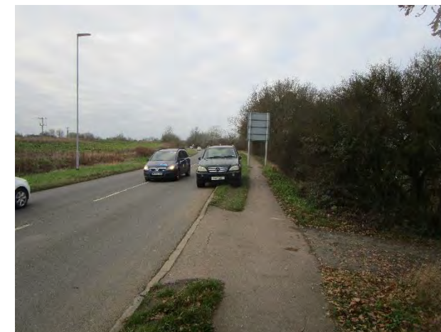
This path is not wide enough and does not have adequate separation from the carriageway and highway space needs reallocating. Measures may be needed to prevent parking like this.
