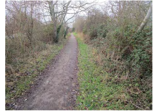
This path needs widening to 3m and to be designated as cycling only. Careful design to protect ecology is needed.
