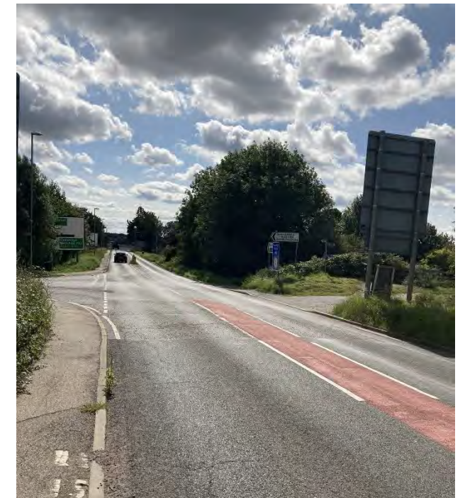
Fig 7.2.4.1 View of Station Road looking towards the Queen Adelaide Way junction.
