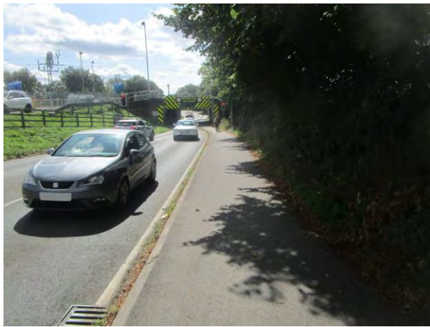
Fig 7.2.3.4 View towards the railway from near Ely Station entrance.
