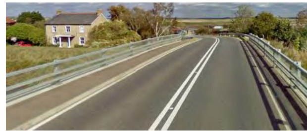
Figure 7.2.8.1 Existing River Lark bridge
