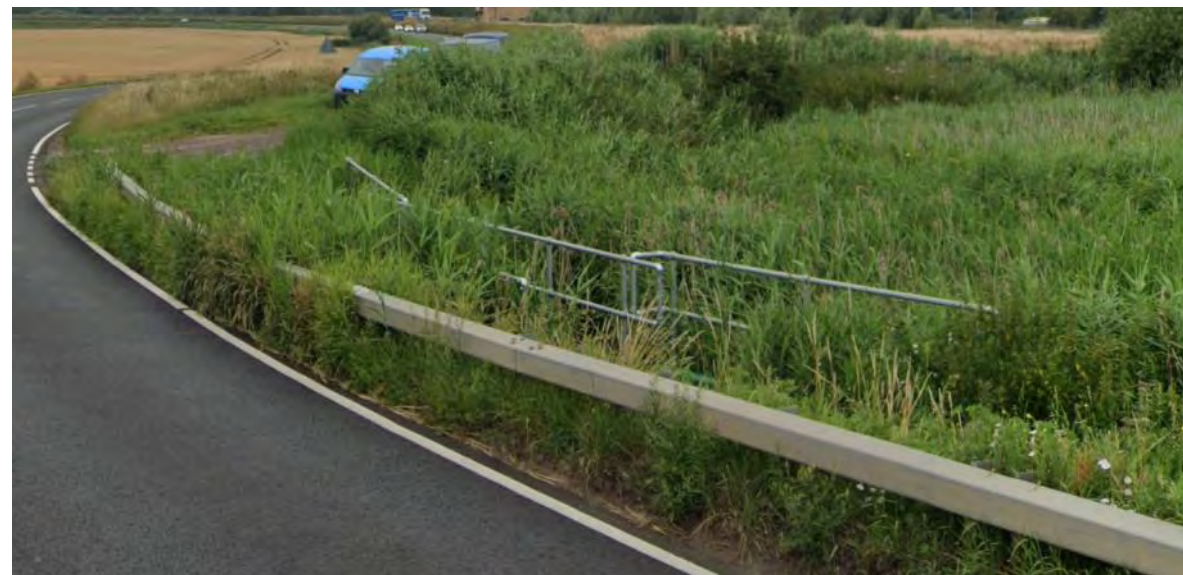
Figure 7.2.5.2 Pedestrian bridge over water course
