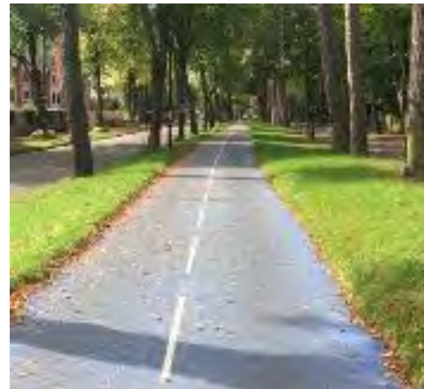
Figure 3.5: Smooth, tarmac surface, accessible for all non-motorised users (Photo: Sustrans)
