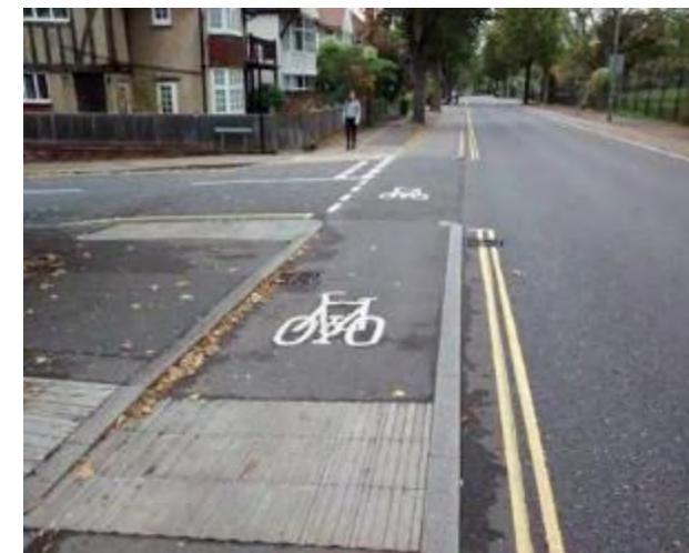
Figure 3.2: At grade crossing of side road with separation for traffic, cyclists and pedestrians (Photo: Sustrans)
