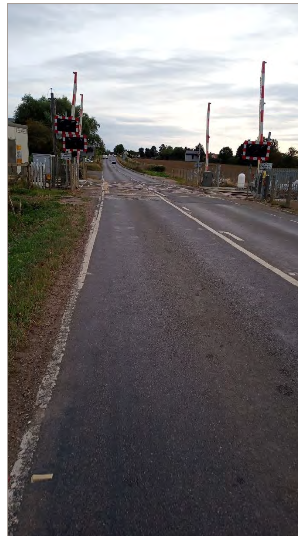
Figure 7.3.4. Approach to the level crossing from Littleport. No changes are proposed for the railway infrastructure.
