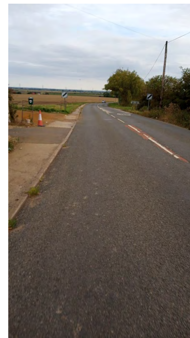
Figure 7.3.5. View towards Chettisham and Ely. Marked cycle lanes in compliance with LTN 1/20 should be considered, along with the removal of centre lines and changes to the speed limit.
