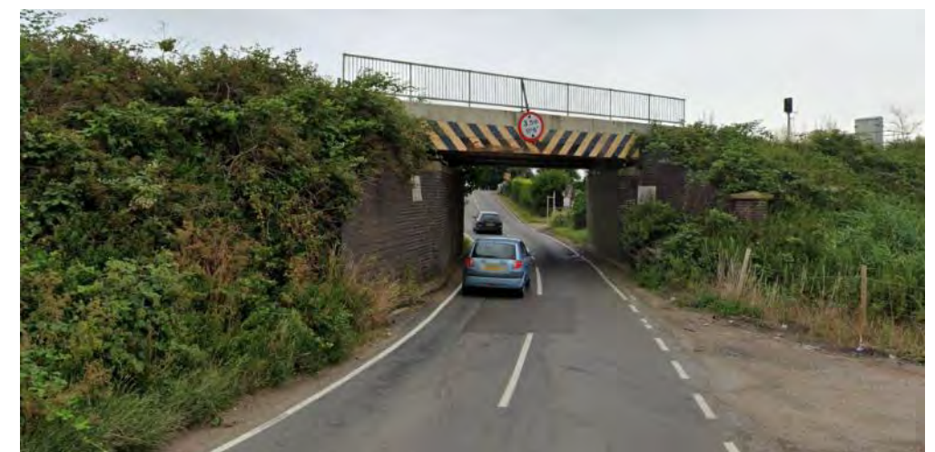
Figure 7.2.6.1 Existing railway crossing with limited space.
