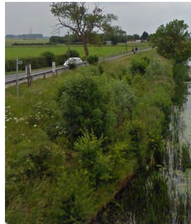
Figure 7.2.9.1 Branch Bank from Victoria Street
