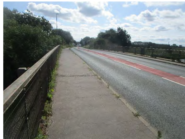
Fig 7.2.3.5 View towards Soham of Station Road showing the existing shared use provision and low parapets.
