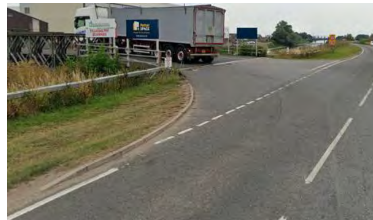
Figure 7.2.5.3 Quarry side road showing barriers.
