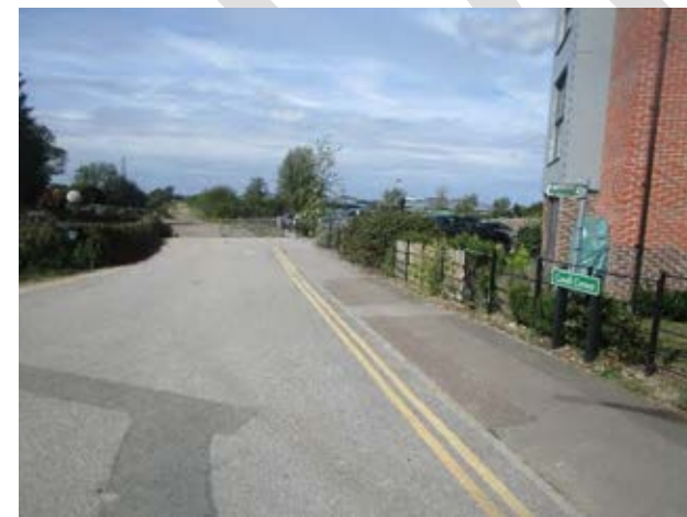
Fig 7B.11.1 View of Covell Corner and the public footpath that runs alongside The Shade Primary School.
