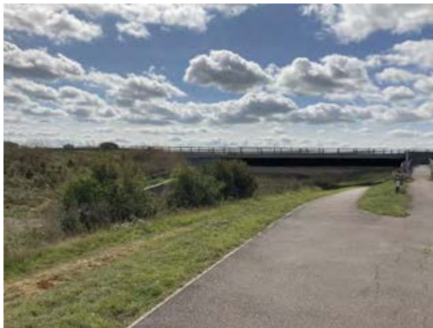
Fig 7D.5.1 - image showing path under bypass from Stuntney Causeway side.
