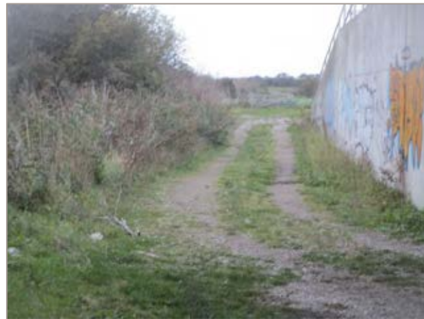
Fig 7D.5.3 – view of track and bypass structure from opposite side of drain to path.
