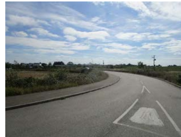
Figure 7C.24.2 View of The Shade Primary School access road. The route can follow the road and would need a new path to the right to link with the existing path along the school boundary that leads to Covell Corner.
