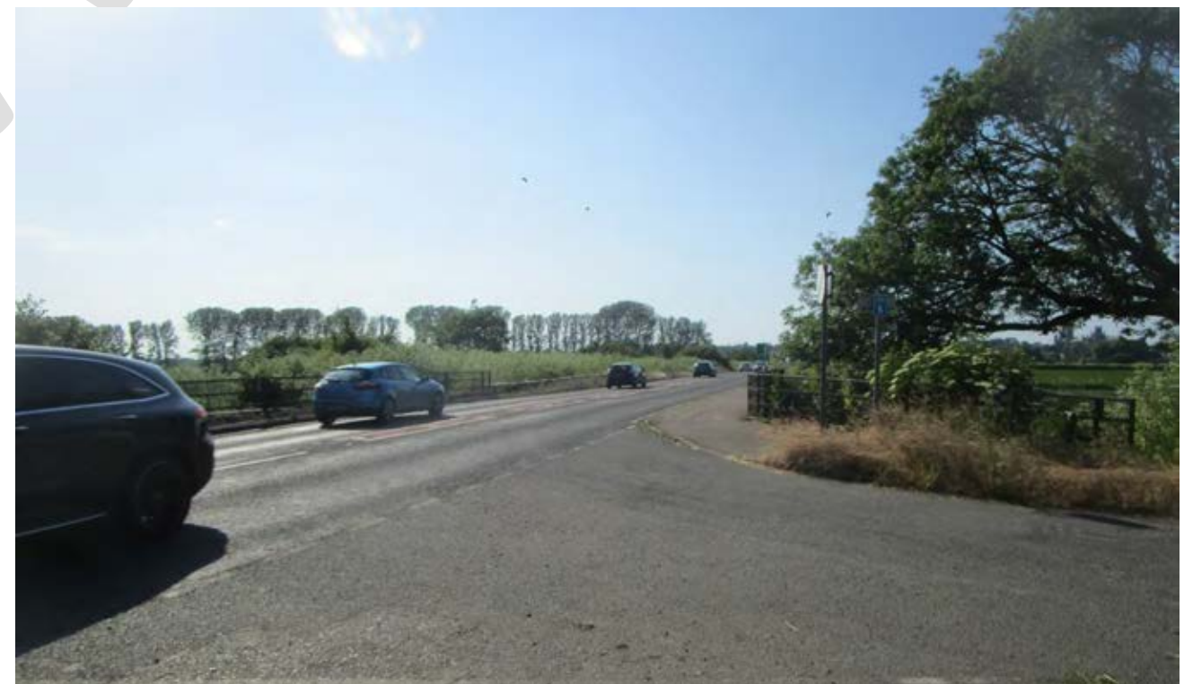
Fig 6.6.2 showing the A 142 - a particularly difficult road to cross on foot or bike due to the high speeds and steady flow of traffic.
