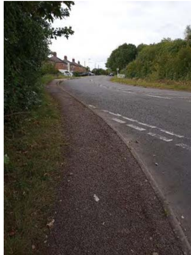
Fig 7C.4.5 View of Soham Road, from the A142, where the ramp would need to cross over the road and then be on the right.
