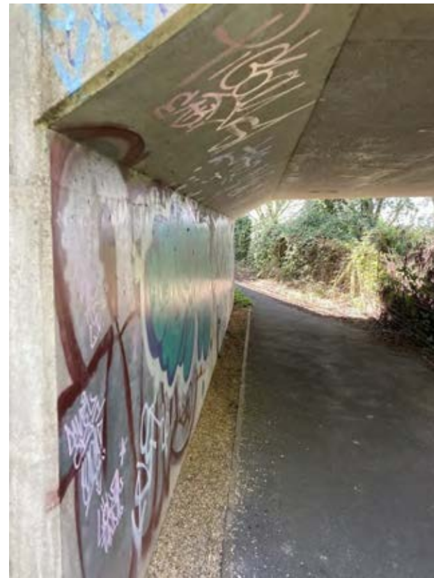
Figure 7D.7.2 Image showing path under railway with stony verge.
