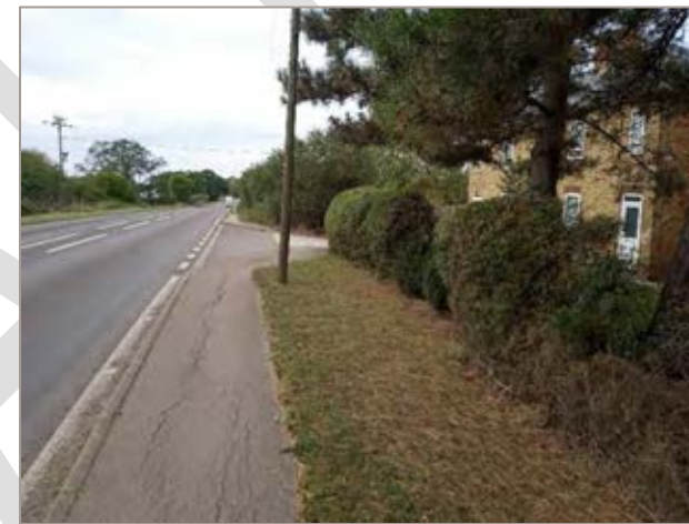
Fig 7C.9.1 There is not sufficient space for a route to pass between residential properties and the A142 unless major works were carried out to realign the carriageway. Options on private land set away from the road appear to be better.
