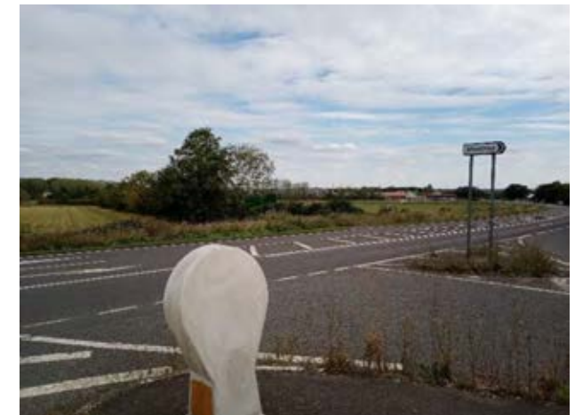
Fig 7A.7.1 View of the A142 at the Stuntney South junction
