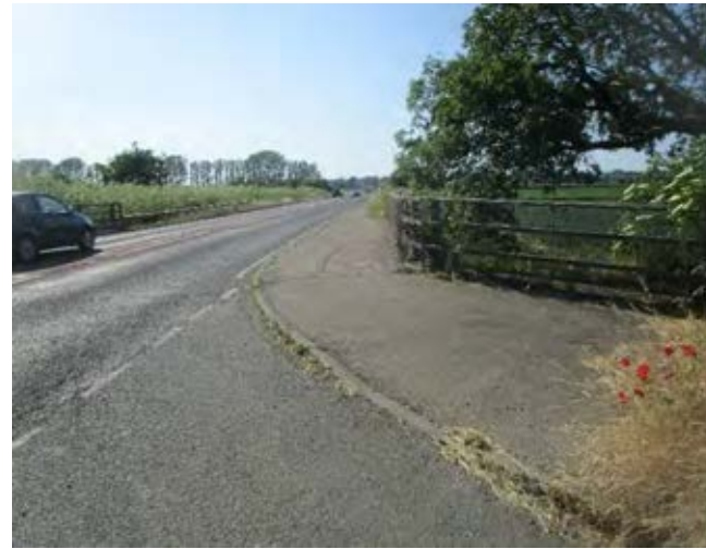
Fig 7A.4.2 The existing crossing.
