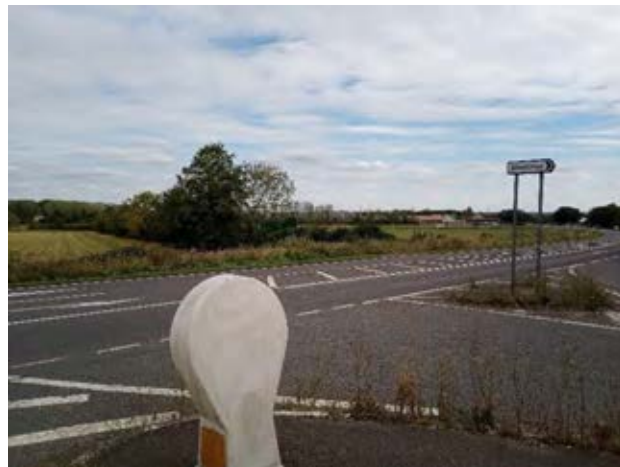
Fig 7A.1 View of the A142
