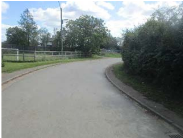
Figure 7D.14.1.- Barway Road in the village
