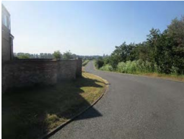
Fig 7G.4.1 Image showing view of Stuntney Causeway view towards Ely.
