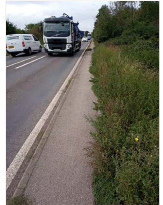
Fig 7C.9.2 The aim of options outlined in vii, viii and ix is to find a suitable alternative to this path, which is the best option currently available, and which does not extend to Ben's Yard entrance.
