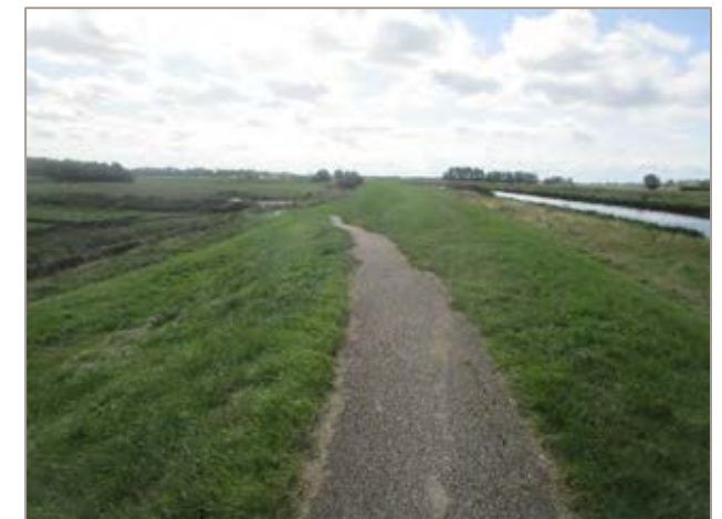
Figure 7D.9.1 Image showing the existing ramp.
