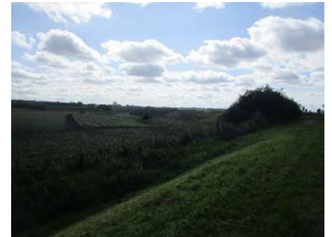
Fig 7D.6.1 - image looking towards railway showing foot of embankment.
