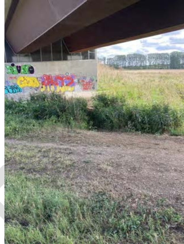
Fig 7D.5.4 – view of bypass structure.
