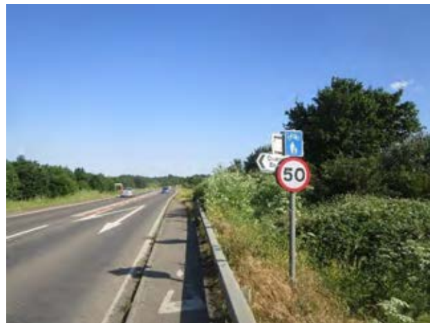
Fig 7A.4.1 The existing path
