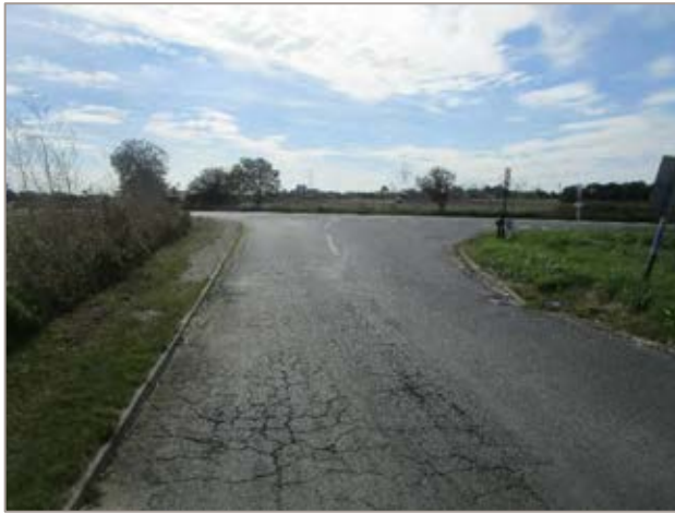
Figure 7C.23.2 View from Barcham Road of the junction showing the wide junction which could be tightened up.
