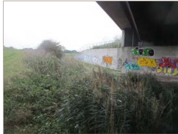
Fig 7D.5.2 - image showing bypass and track that goes under bypass beside the drain.
