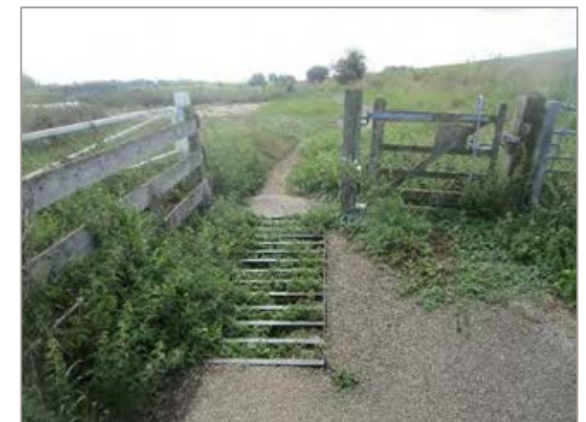
Figure 7D.9.2 Image showing the existing cattle grid.
