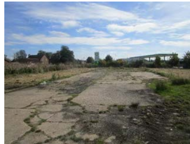
Fig 7B.4.2 View towards the BP service station with the A142 on the left. The route would have to turn left to follow the boundary to join the service road seen in Fig 7B 4.3.
