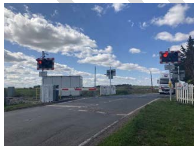
Fig 7D.20.1.- Image showing level crossing.
