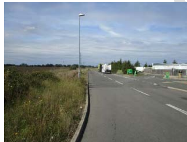
Fig 7B.4.3 View back towards Rosefield House showing the Service Road behind the BP service station where a link with the path in Fig 7.4.2 would be needed.
