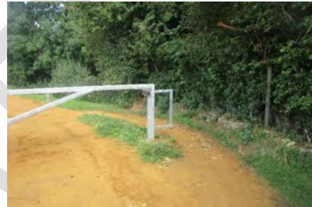
Figure 7D.12.1 Image of gate and bypass from Barway side.
