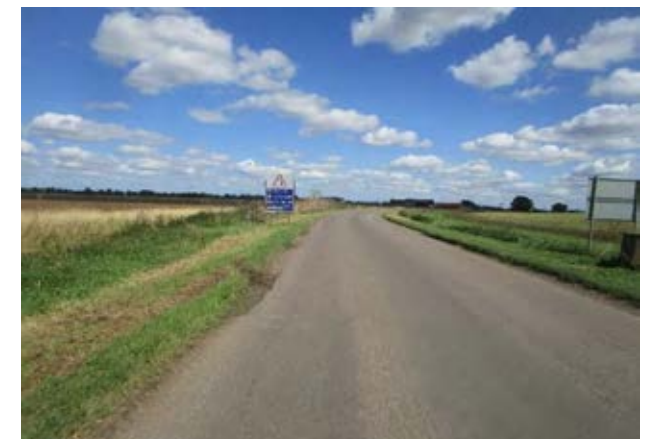
Figure 7D.17.2 - Barway Road with space besides the road for a new path set away from the carriageway.
