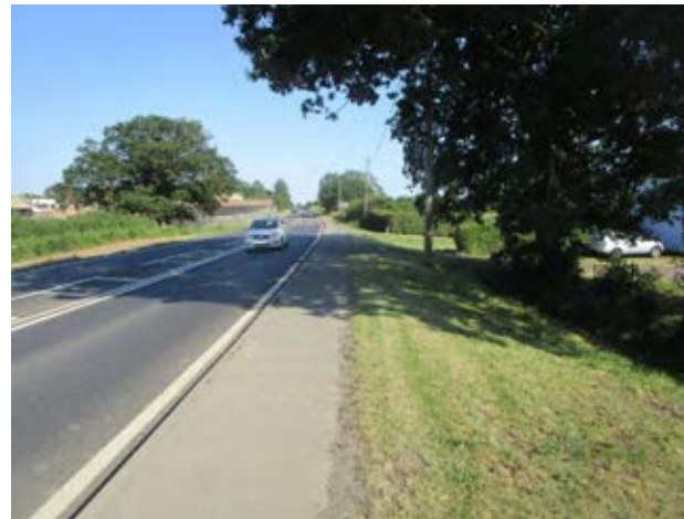
Fig 7A.8.2 View of the A142 from near Ben's Yard
