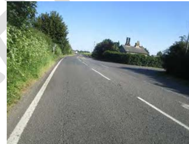
Fig 7A.8.5 Property and very limited verge space at the Barway Road junction.
