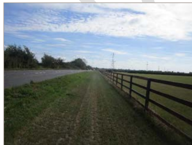
Fig 7B.3.1 The fence is likely to need to be moved back slightly here to get sufficient space for a path.
