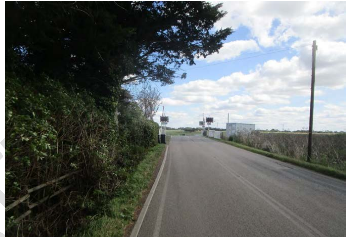
Fig 6.6.1 Existing level crossing on Barway Road
