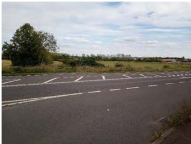
Fig 7C.4.3 View of the field and potential bridge ramp site from Stuntney towards Ben's Yard.
