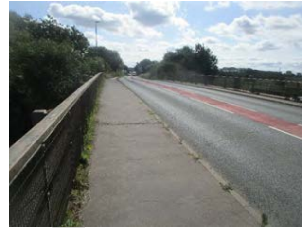
Fig 7A.1.7 View towards Soham of Station Road showing the existing shared use provision and low parapets.
