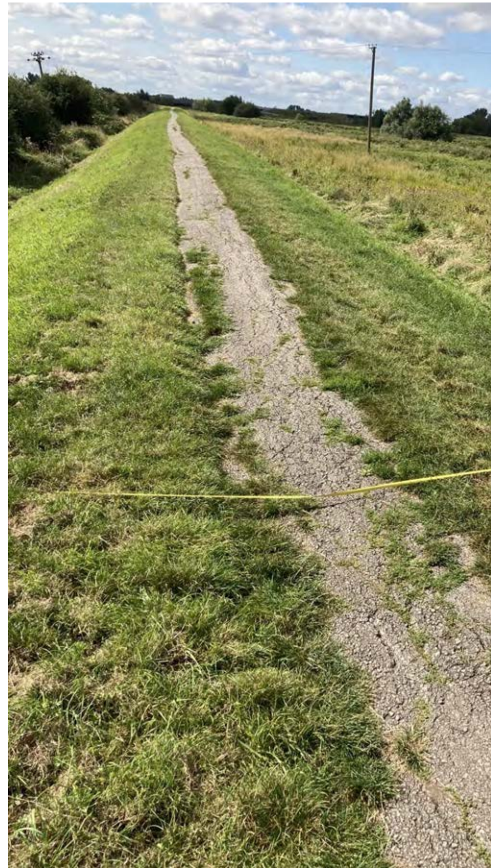
Fig 7D.4.1- image of existing path with a tape showing 3m.
