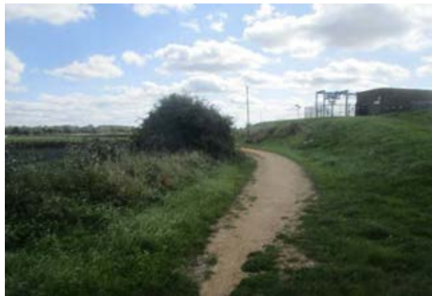
Figure 7D.10.3- showing the existing path.
