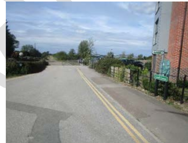
Figure 7C.24.3 As with Option B the route would enter Soham via the track along the school boundary and through Covell Corner.
