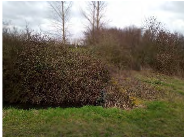
There are some existing culverts to cross the watercourse to link with the byway and using these would be a good option.
