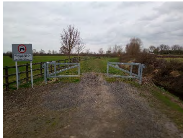
The start of the byway (left) at the southern end. It is suggested that this remains unchanged.
