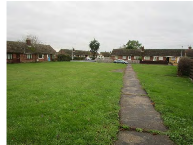
Existing path from Fordham Road, Soham towards Cornmills Road. In this area new segregated cycle paths and footpaths are needed.
