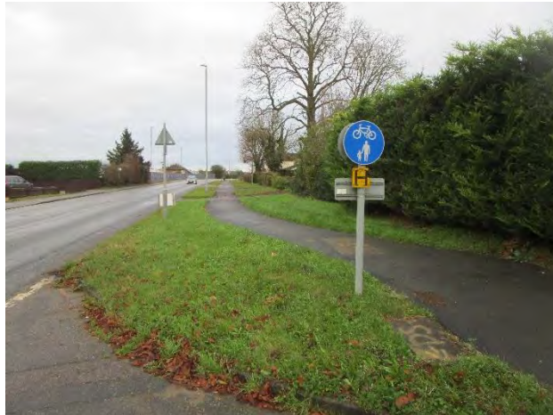
The current standard of cycle provision in Soham is not LTN 1/20 compliant and the network is incomplete.
