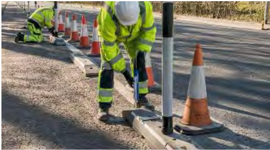
Photo: Rosehill Highways showing segregated cycleway being established on existing carriageway.
