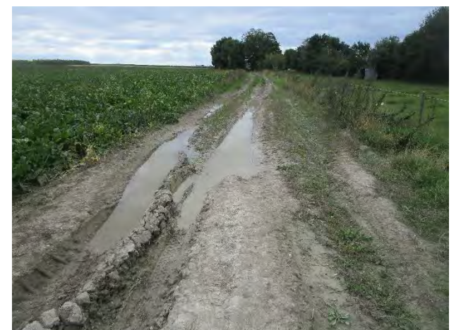
The byway is in poor condition and would need major work.
