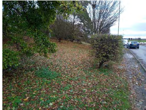
There is space for a segregated path away from the carriageway, but it will need surveying and landowner's agreement.
