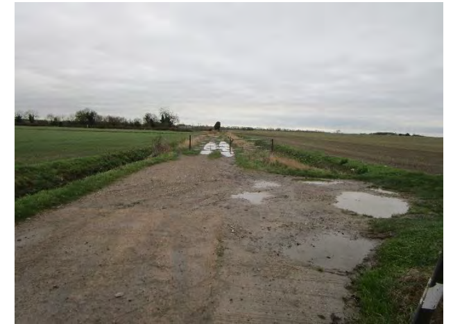
View from Ness Road along byway towards disused railway (iv on following plan).
