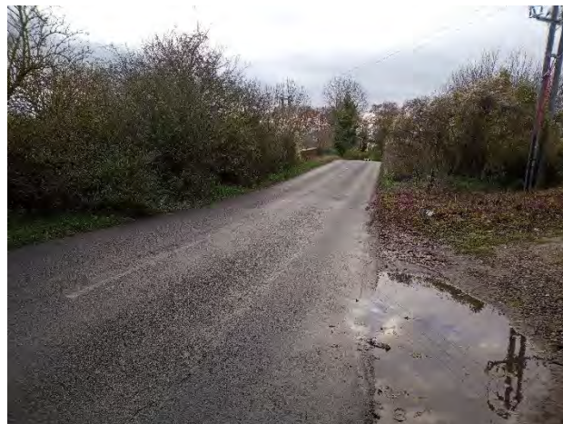
View towards the railway bridge from near the Turners entrance. A potentially quiet lane linking with a major industrial road.
