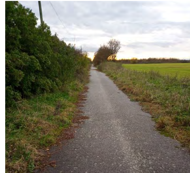
The former road is in good condition and is a right of way to the east of the A142 making this an obvious access to/from Fordham.
