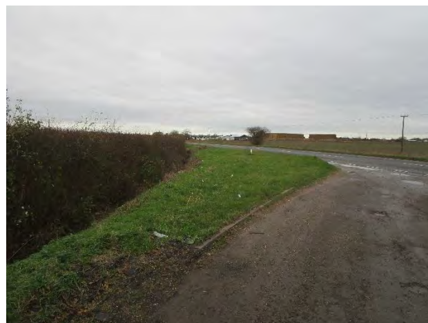
Approximate position for a new bridge over the B1102 (note the overhead power lines, which would need moving.)
