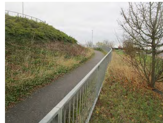
Existing ramp to existing bridge over A142. There is space to widen the path and move the fencing back from the path or remove the fencing all together.
