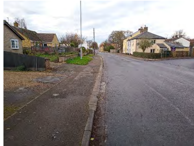
The River Lane/ Market Street/ Newmarket Road junction will need careful design and is the area where segregated cycleways would meet.
