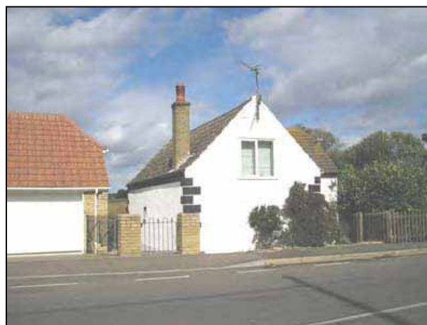
Building lower than present road surface
