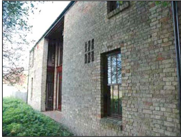
Converted barn, adjacent to Back Lane
