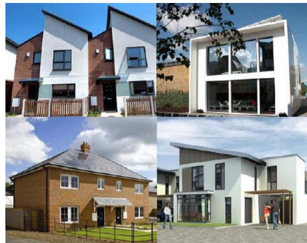
Examples of schemes in a variety of architectural styles which are already meeting Levels 5 and 6 Code for Sustainable Homes – www.zerocarbonhub.org Clockwise from top left: Astling Green, Blackpool: Level 5; The CUB Modular Home, Watford: Level 5; Miller Homes Miller Zero Housing Project, Basingstoke: Level 6; Brookwood Farm, Woking: Level 5.
