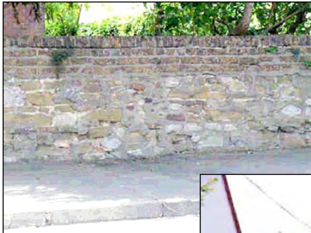
Left: St John's Wall from Cambridge Road
