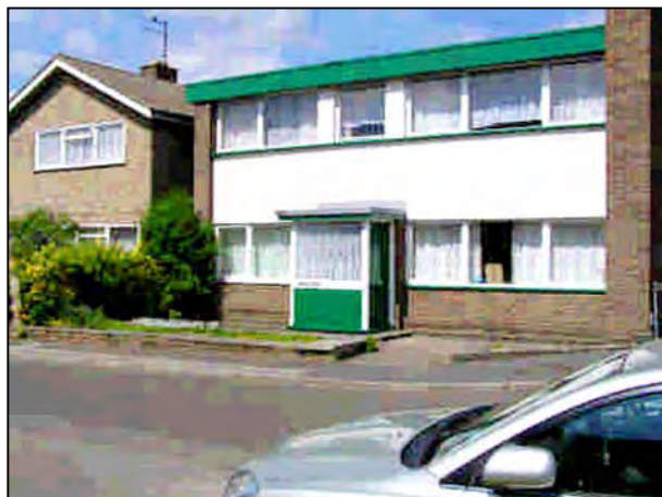
Unsympathetic building on West End
