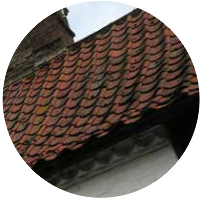
CLAY PANTILE ROOF
