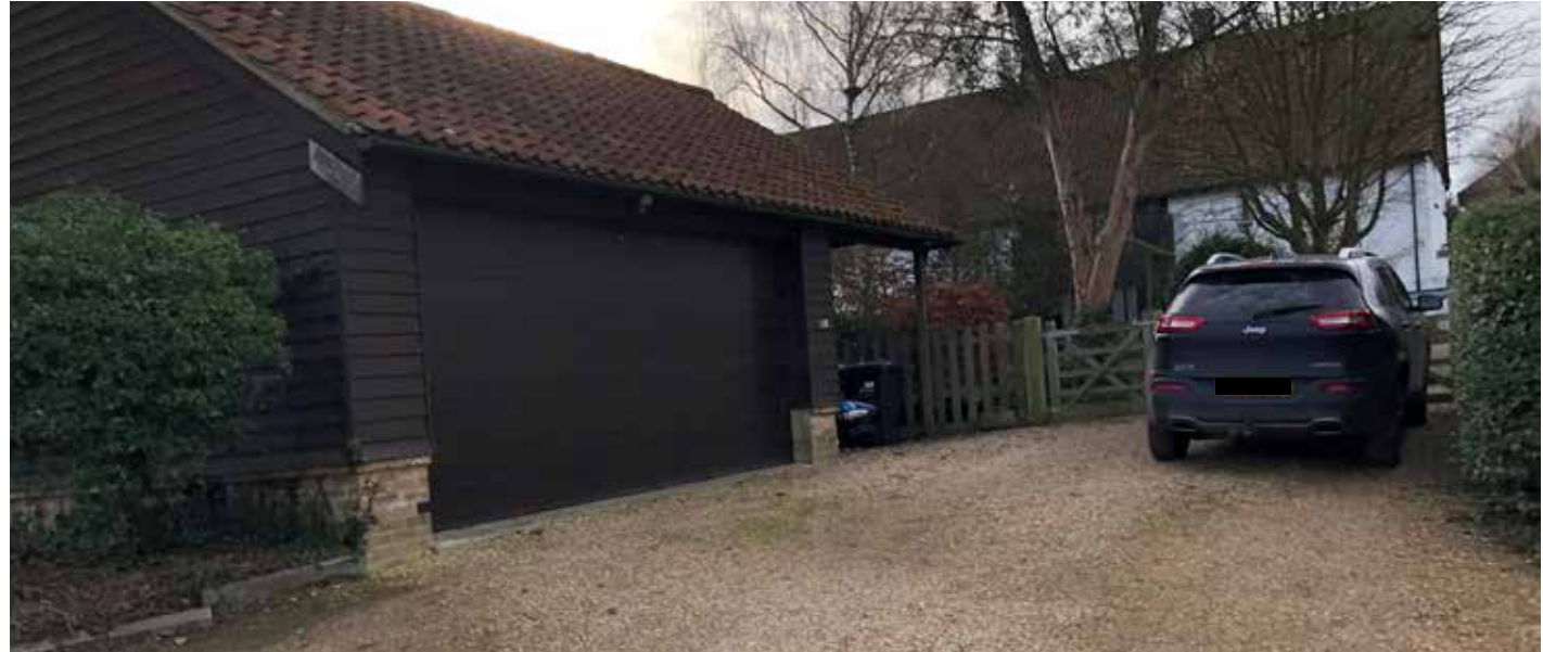
Figure 41: House with front yard parking and garage (left) built with traditional materials found in Reach - pantile roof, black weatherboarding, and yellow brick (Burnwell whites). Note: it is recommended that garage structures are set back from the building line.
