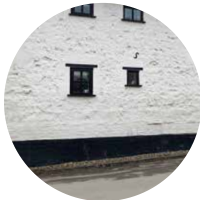
BLACK-PAINTED BUILDING PLINTH
