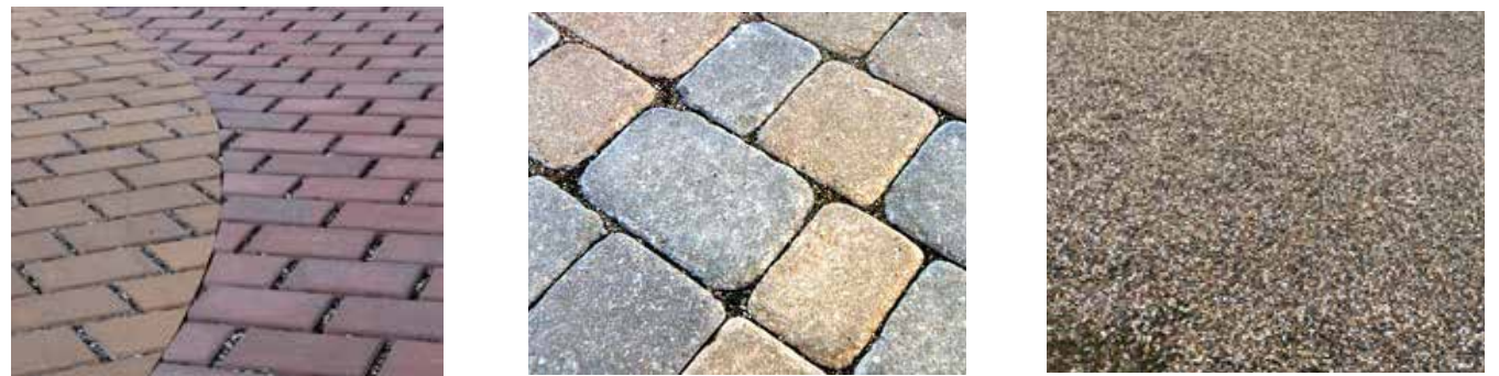
Figure 58: Examples of permeable paving treatments: clay pavers, stone/precast concrete setts, and unbound gravel.
