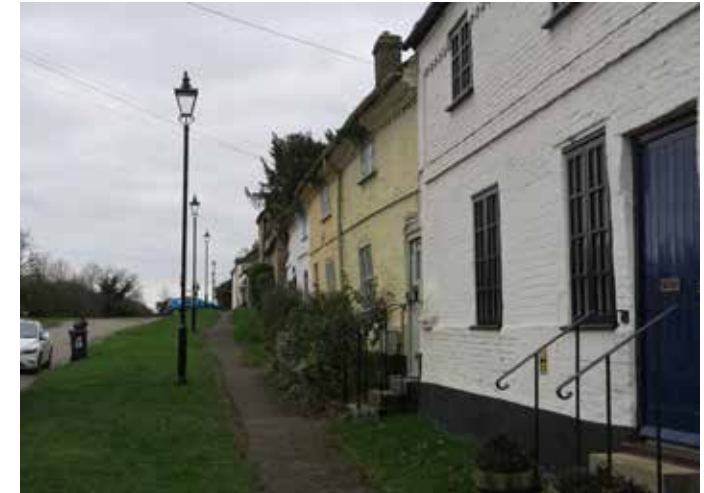
Figure 52: Buildings aligned along the southern side of Fair Green behind a narrow planting strip.
