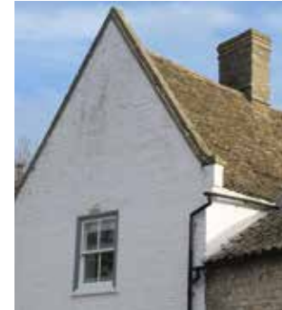
Painted-brick parapet gable.
