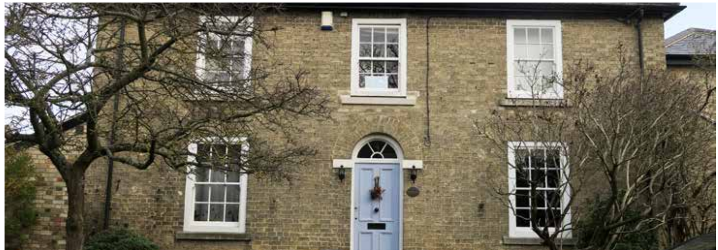
Figure 50: A façade with a simple and attractive arrangement of multi-pane sash windows and fanlight above the entrance door.
