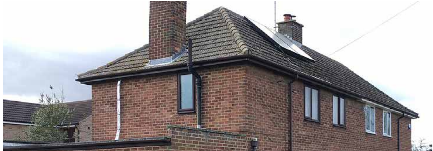
Figure 61: 1950s house on Swaffham Road retrofitted with roof solar panels.
