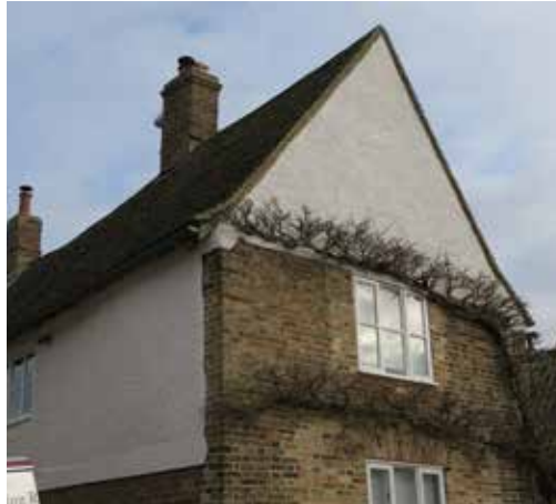
Figure 32: Gabled roof with chimney stacks.
