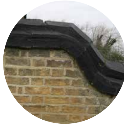
BRICK BOUNDARY WALL
