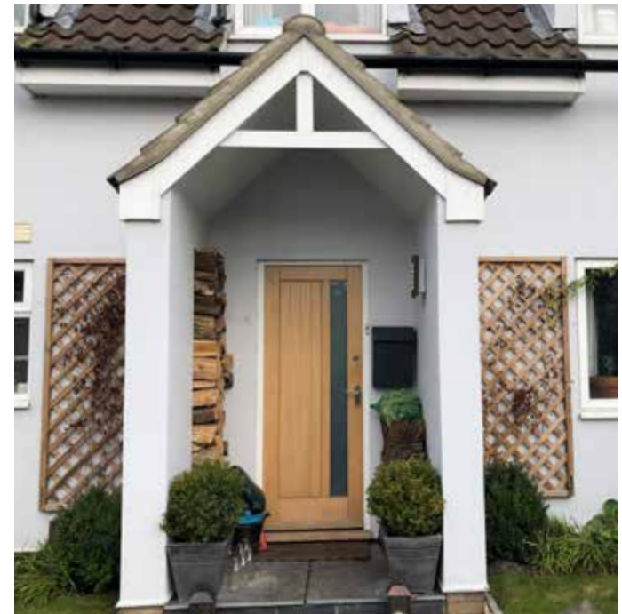
A modern gabled porch with low-level planting to mark the transition between public and private spheres.
