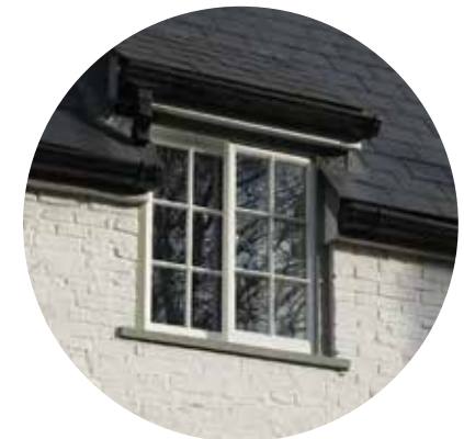
HORIZONTAL (YORKSHIRE) SASH WINDOW
