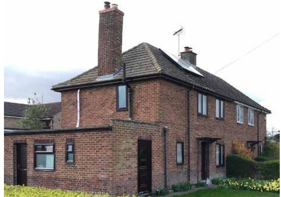
Semi-detached 1920s houses built by the local authority on Ditchfield.
