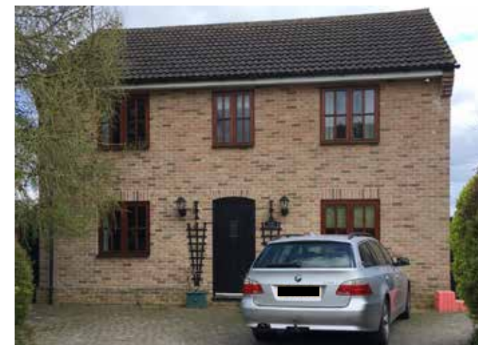
Figure 48: Infill house on Ditchfield that respects the regular layout and roofline of the adjacent two-story buildings.
