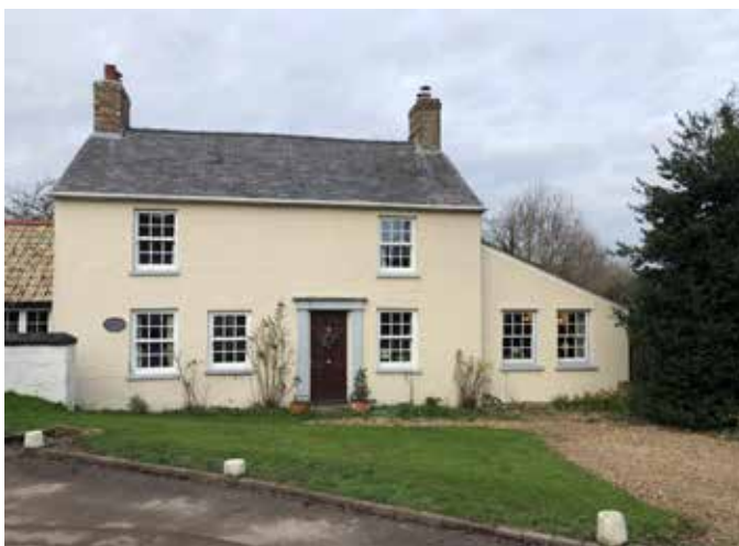
Figure 46: House with a side extension with the same treatment as the main body.
