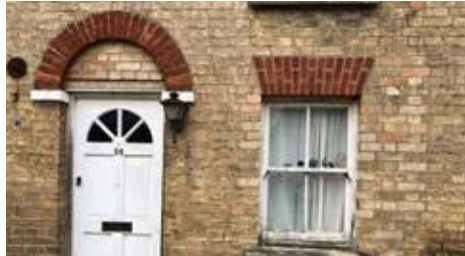
Yellow brick façades known as Burwell Whites with contrasting red brick lintels.
