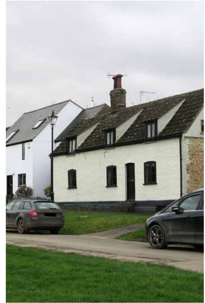
Figure 37: Informal on-street parking on Fair Green, must carefully managed to ensure adequate access by other vehicles, including buses.
