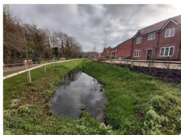
Example of Sustainable Drainage System capturing rainwater run-off
